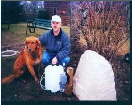
This "Mock Rock" for an attractive, finished look can camouflage the installation of the metering pump at the well.
